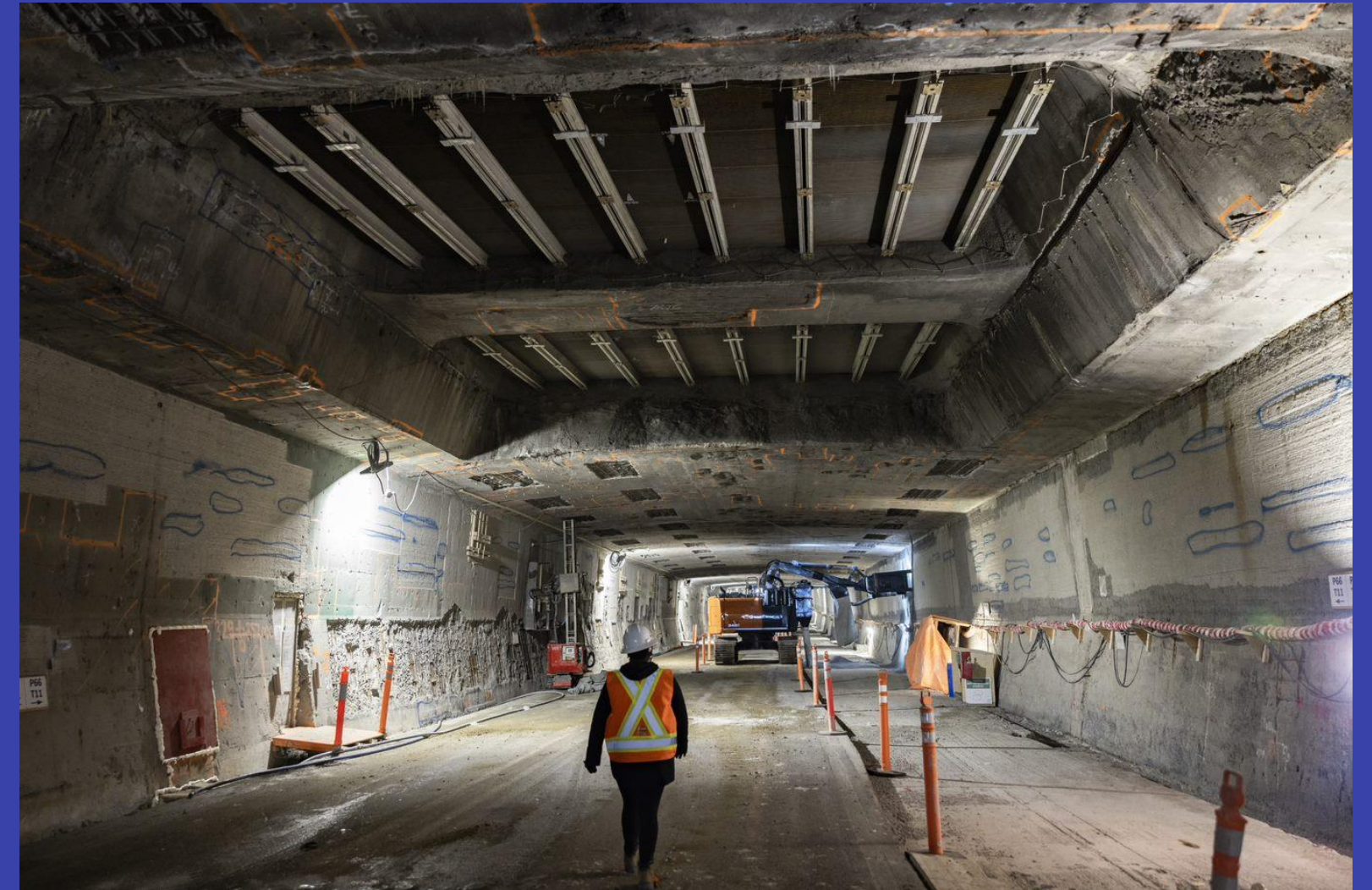
Structural repair work for the southbound tube under the ventilation shaft
